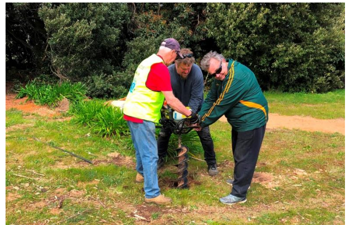
Digging the post holes
