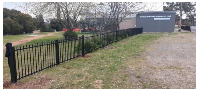
Looking good at the end of Day 1
