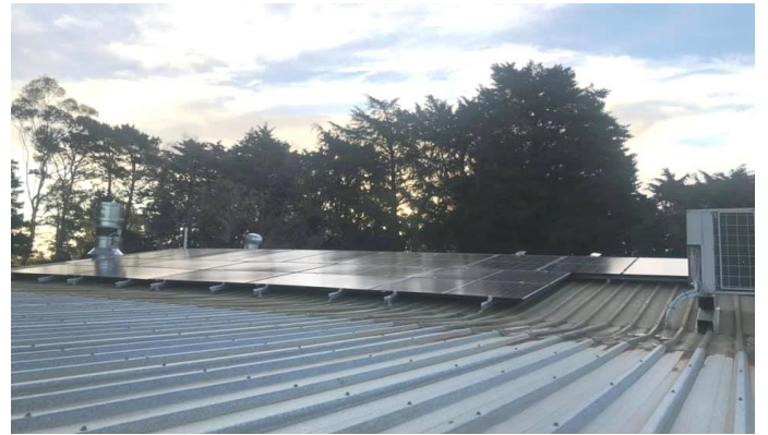
Solar power system installed on clubrooms
