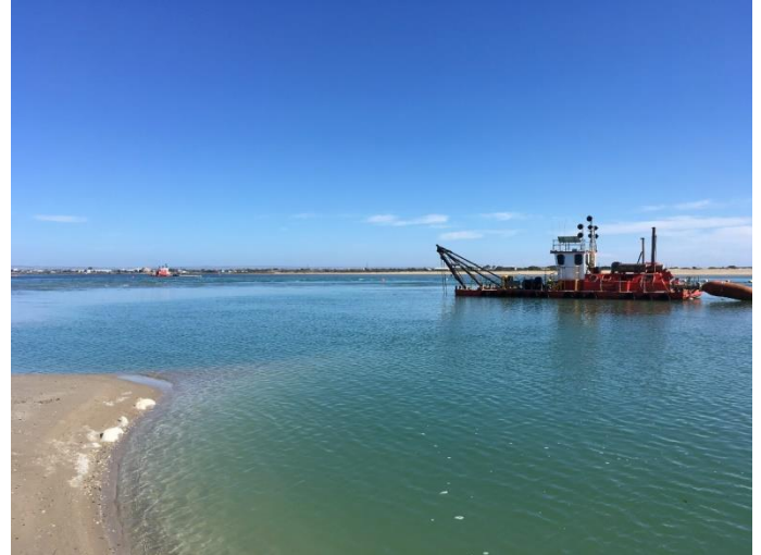
Photo: Dredges at the Murray Mouth.
