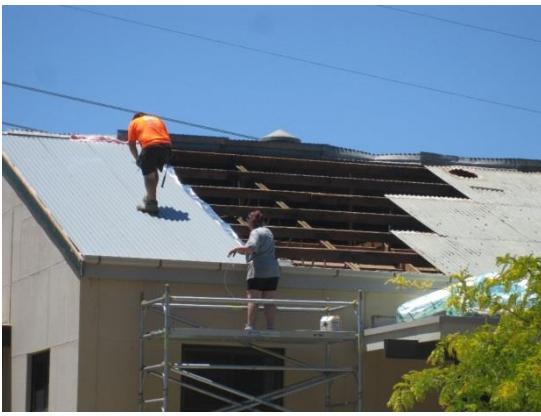
Replacing the roof
