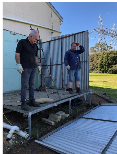
Removing the old attachment.
